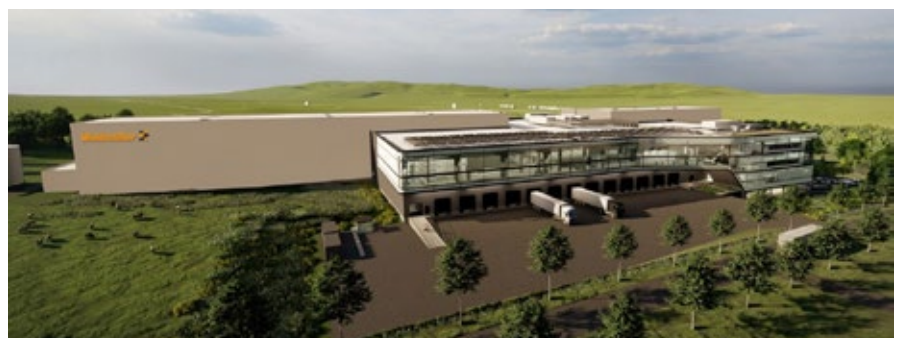
Visualization of the logistics center in the industrial area "Kindel" in Hörselberg-Hainich. Photo: Weidmüller
