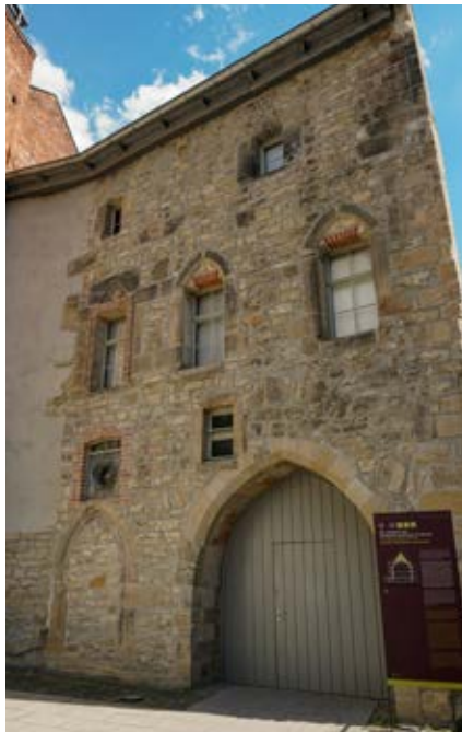
North façade of the Old Synagogue in Erfurt's old town. Photo: www.unesco.de/pressefotos – © Pro Denkmal
